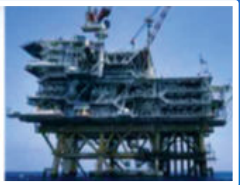
Offshore Oil Platform
